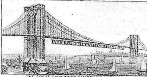
THE GREAT EAST RIVER SUSPENSION BRIDGE.
